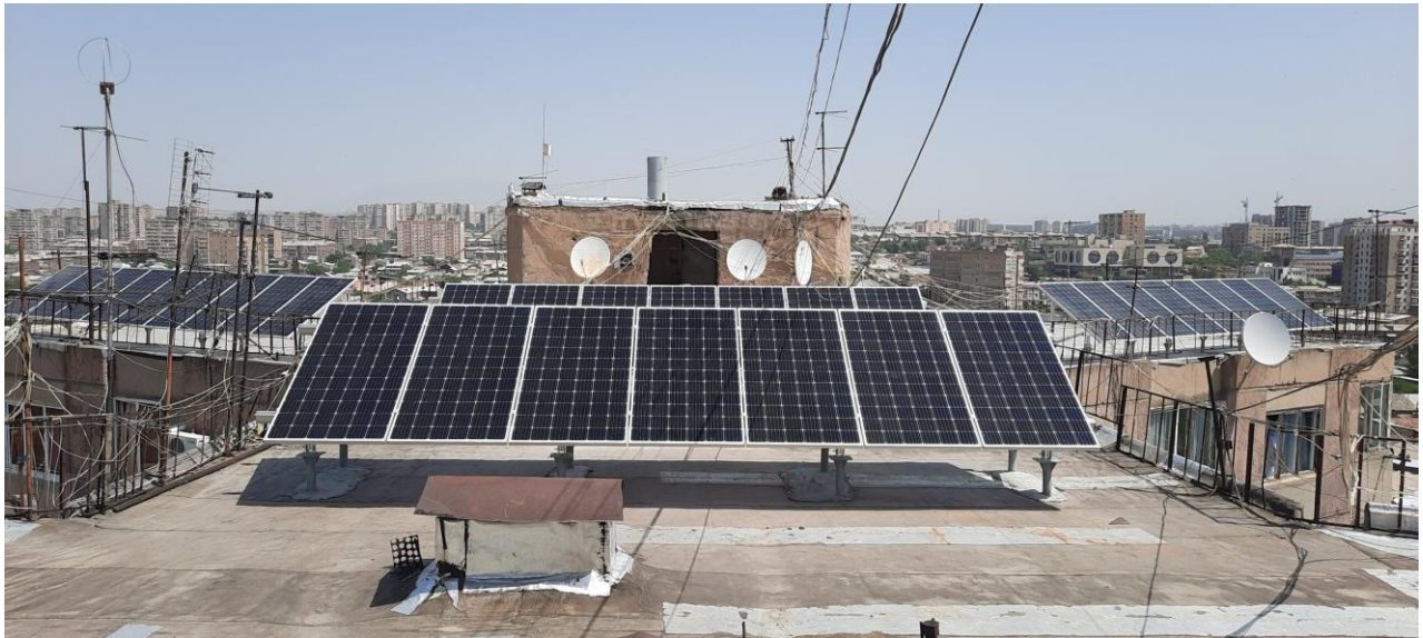
Fig. 1. EU4Yerevan-Solar Community Project. Solar PV system installed on the roof of multi-story residential apartment building. https://com-dep.eu/eu4yerevan-solar-community-project-promotes-renewable-energy-energy-efficiency-retrofits-in-multi-apartment-buildings/
